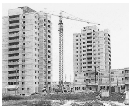
Place Bardy en construction, 1970
